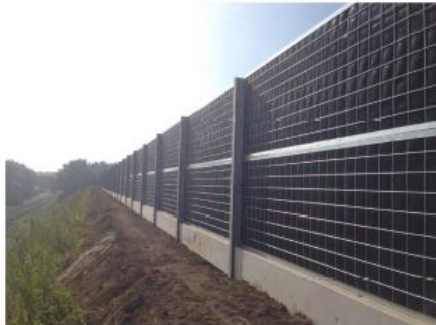
Noise-Reducer geluidscherm Type SA-80 H=4,5m, hok 4m
